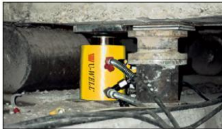
Replacing adjustment rolls under a fly-over with CLRG cylinders, for controlled lifting and lowering.
