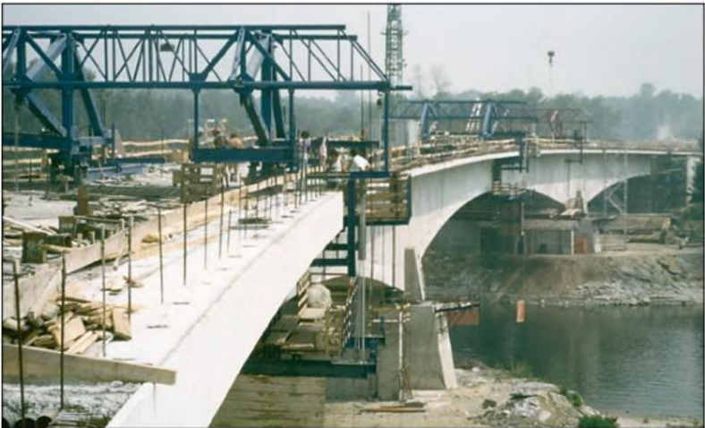
在這一立交橋中，CLL油缸用來支撐混凝土梁，調平支座並將4000噸的滑動軸承置于橋墩與支座中間。 For this curved bridge, CLL-cylinders were used to support the concrete beams, to level the pierhead and to place 4000 ton slide bearings between pier and pierhead.
