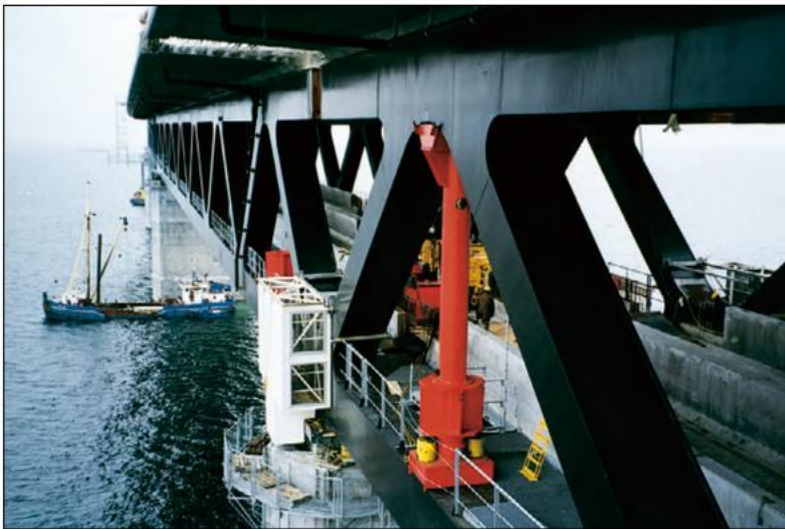
Replacing adjustment rolls under a fly-over with CLRG cylinders, for controlled lifting and lowering.
