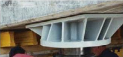
CLL cylinder, mechanically locked, after positioning the curved bridge.
