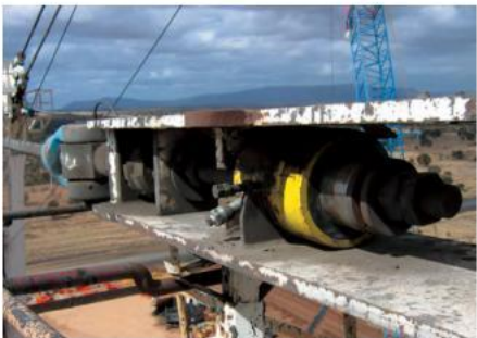
中空柱塞油缸RCH-1003在噴杆吊架安裝中的運用。 Hollowplunger cylinder RCH-1003 used in an application for intermediate boom suspension on a dragline
