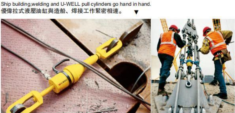
TO lift a load bearing mast into place, BRP-series cylinders were used to tension the supporting cables.
